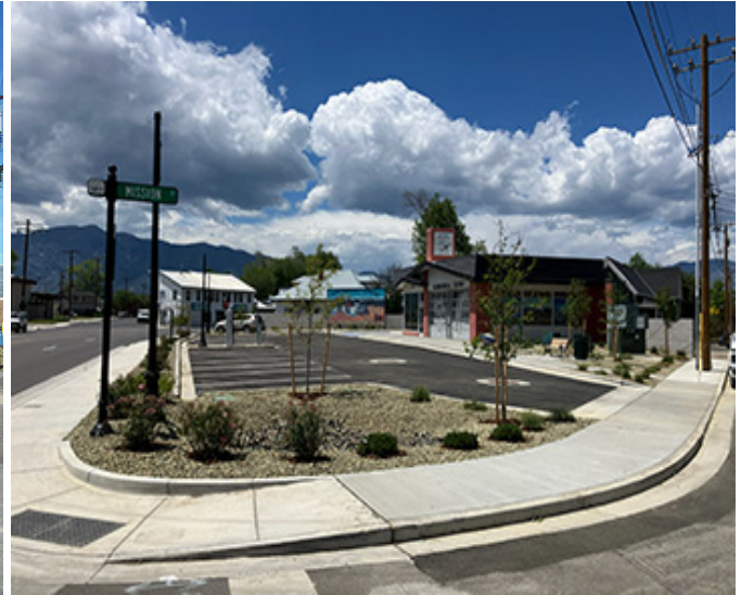
Gardnerville Station after
