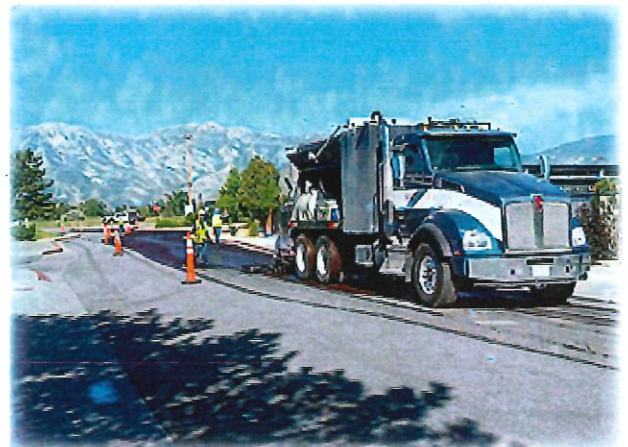
Slurry Seal
