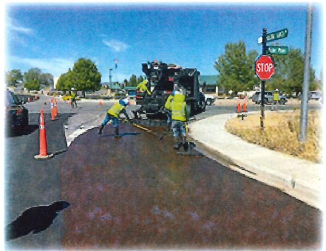
Slurry Seal
