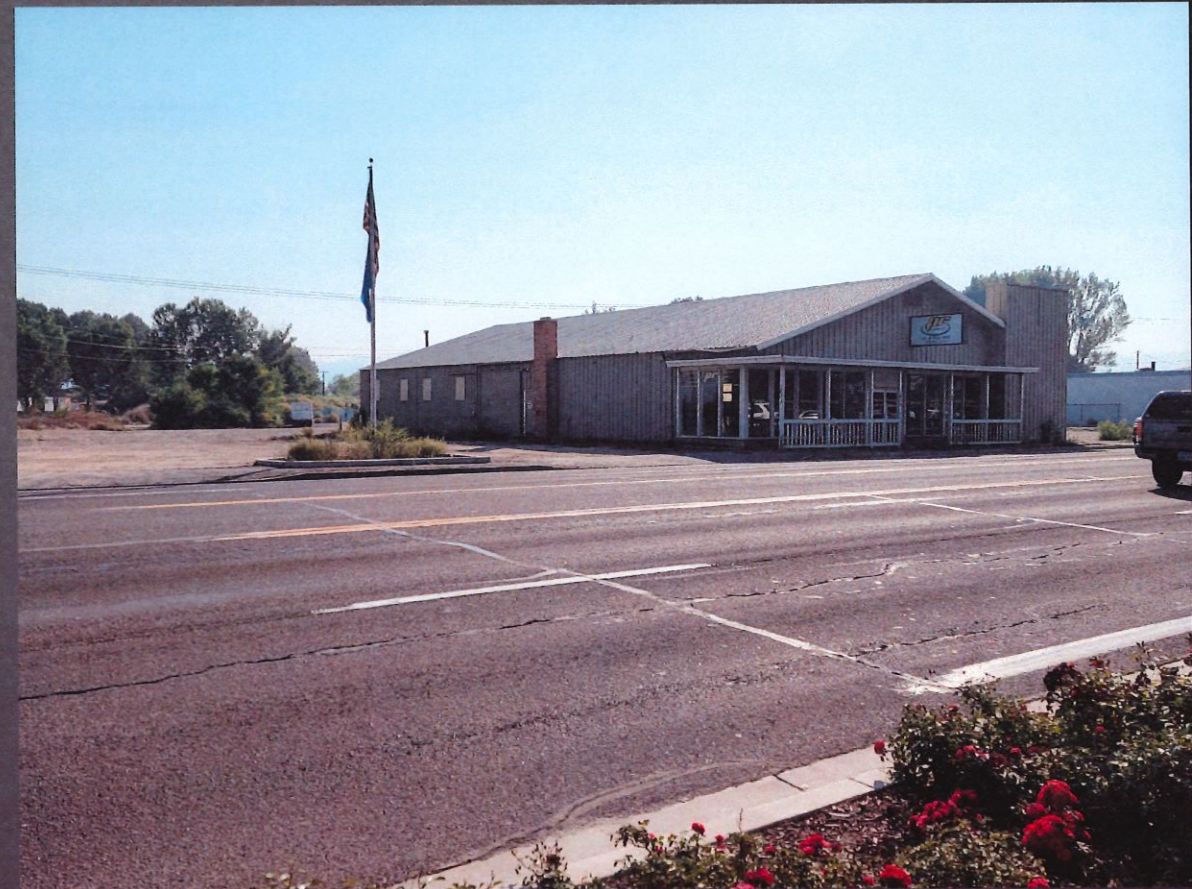
PR SUPPLY, HWY 395, GARDNERVILLE
