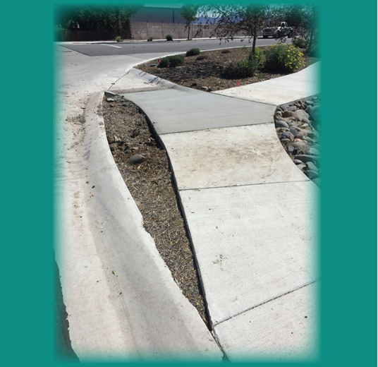
Town Concrete Project
