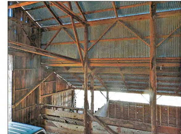
BARN CENTER- NORTH-EAST CORNER (P12 S4.1)
