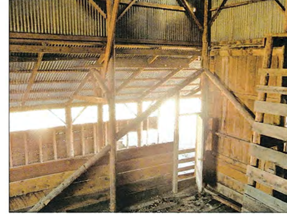
BARN CENTER- SOUTH-EAST CORNER (P3 S4.1)
