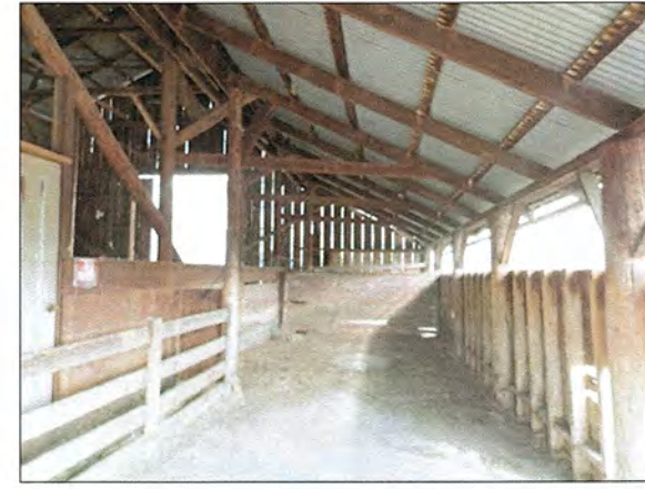
EAST SIDE UTILITY ISLE LOOKING NORTH (P4 S4.3)
