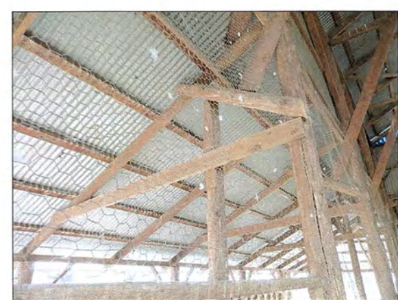
LOW/HIGH ROOF TRANSITION- EAST SIDE (P14 S4.1)
