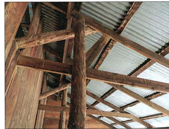
SOUTH END LOW ROOF
