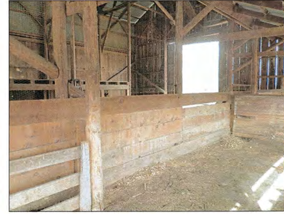
EAST SIDE UTILITY ISLE LOOKING NORTH (P8 S4.3)
