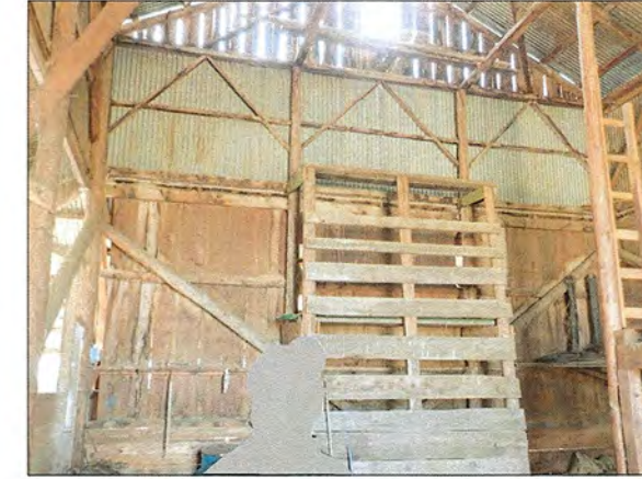
BARN CENTER- SOUTH WALL (P4 S4.1)
