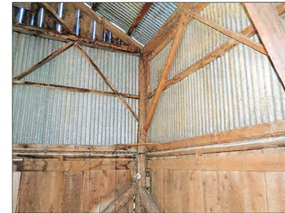
BARN CENTER- SOUTH-WEST CORNER (P8 S4.1)
