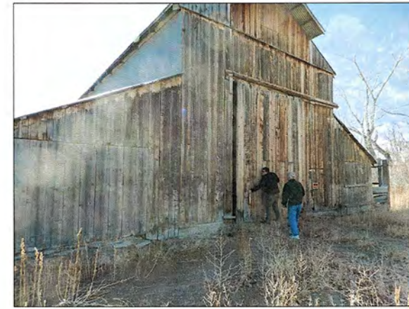
NORTH FACADE (P16 S4.3)
