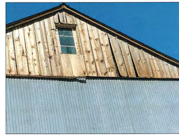
SOUTH GABLE-END (P12 S4.3)
