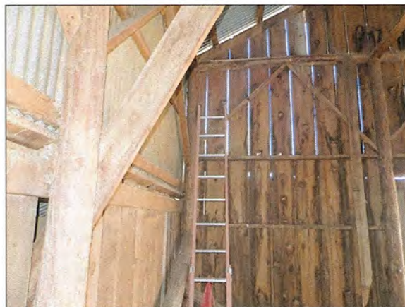
BARN CENTER- NORTH-WEST CORNER (P9 S4.1)
