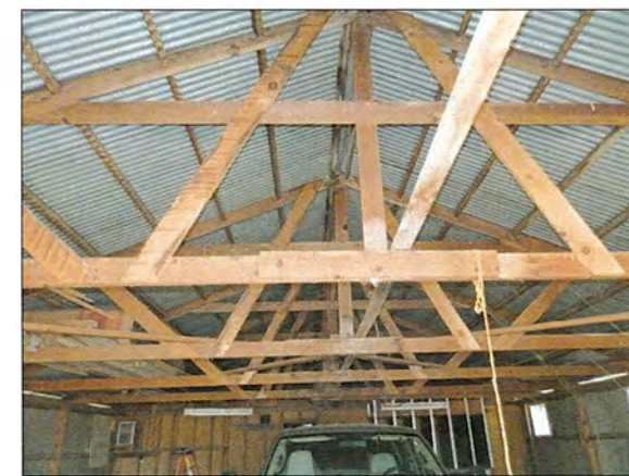
INTERIOR VIEW LOOKING SOUTH
