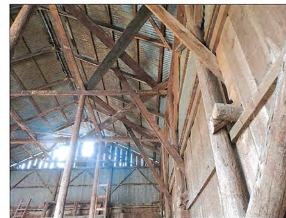
HIGH ROOF AT WEST WALL LOOKING SOUTH (P15 S4.1)
