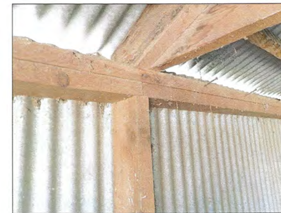
TYPICAL TRUSS OVER STUD
