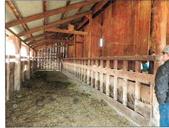
WEST SIDE FEED ALLEY LOOKING NORTH
