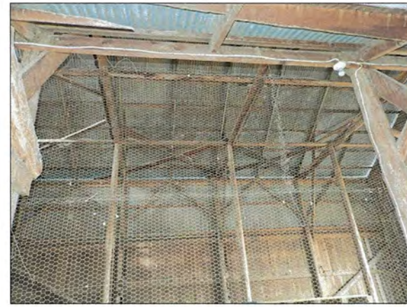
EAST SIDE UTILITY ISLE ROOF TRANSITION (P7 S4.3)
