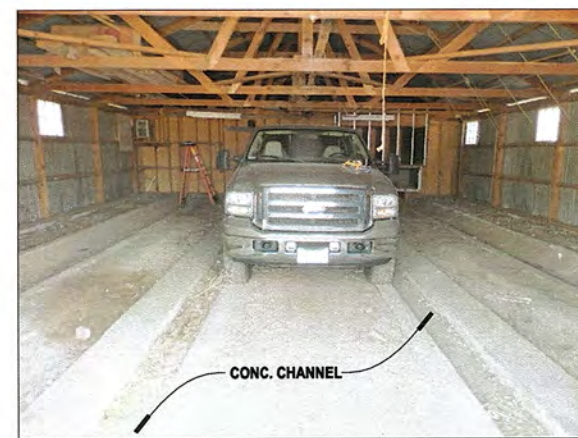
INTERIOR VIEW LOOKING SOUTH
