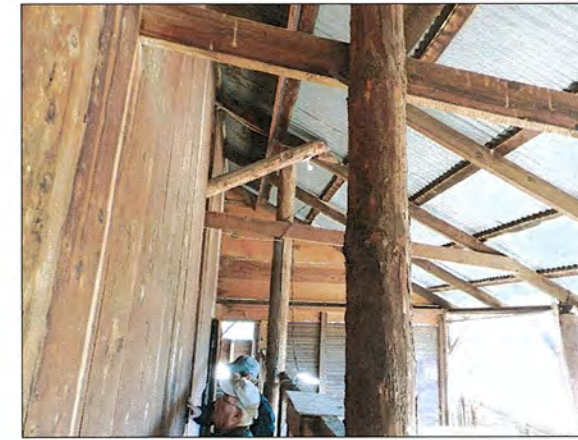
SOUTH END LOW ROOF
