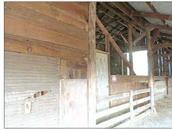
EAST SIDE UTILITY ISLE LOOKING NORTH (P3 S4.3)
