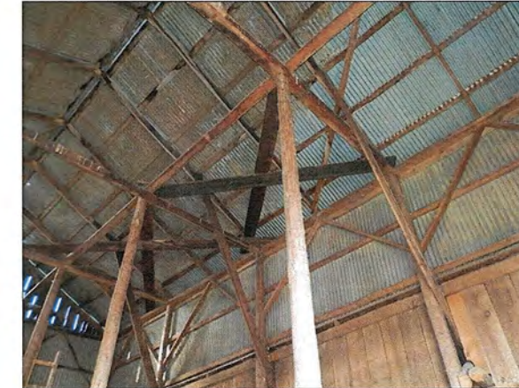
HIGH ROOF AT WEST WALL (P16 S4.1)
