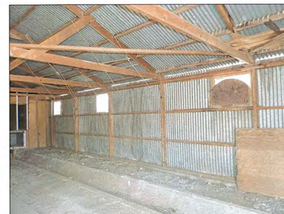
WEST WALL- LOOKING SOUTH
