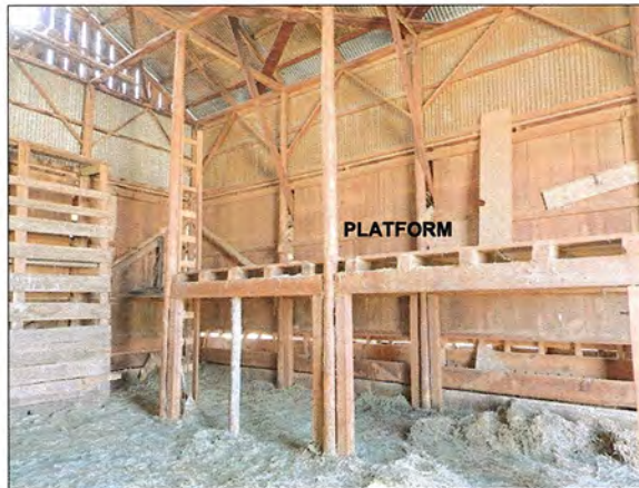
BARN CENTER- SOUTH-WEST CORNER (P5 S4.1)
