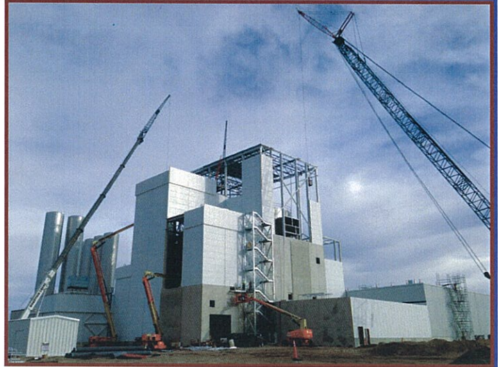
Powdered-milk processing plant in Fallon, under construction.
