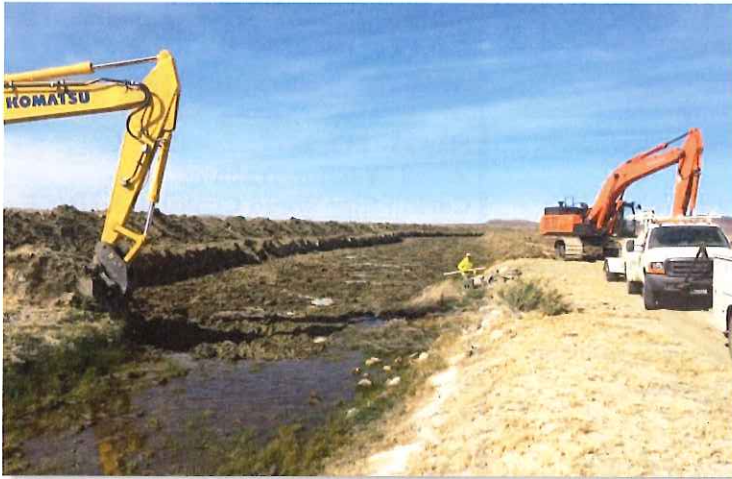
Emergency Bypass being constructed. Photo by: Ernie Schank
