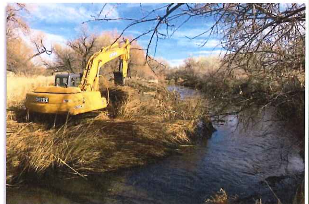
Carson River dredging to remove sediment build-up. Photo by: Ernie Schank
