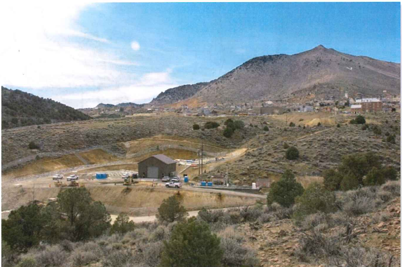
Virginia City and Gold Hill Wastewater Treatment Plant (WWTP) Photo by: Farr West Engineering
