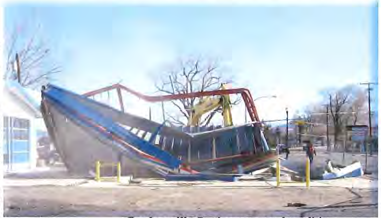
Gardnerville Station canopy demolition
