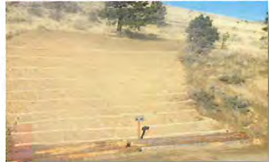
Ash Canyon Restoration Site 1—Erosion Control Photo by Richard Wilkinson
