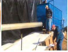
Hopper With Outlet Pipe Leading To Area Inlet
