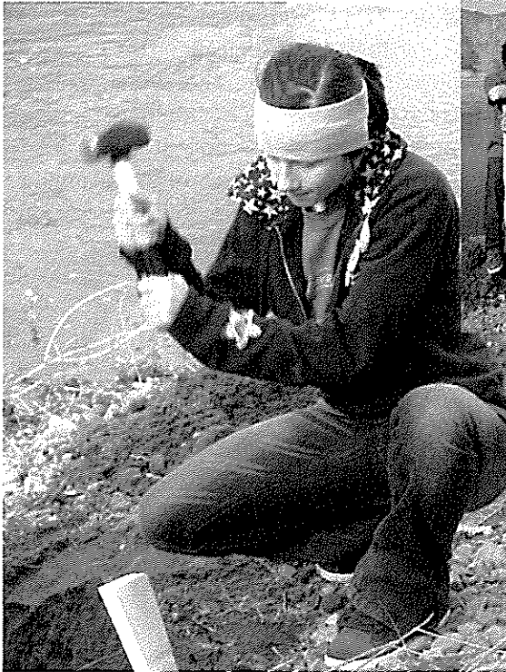
Jennifer Harris stakes willow bundles to the stream bank at Conserve Carson River Work Day 2012. Photo Courtesy of Nevada River Wranglers
