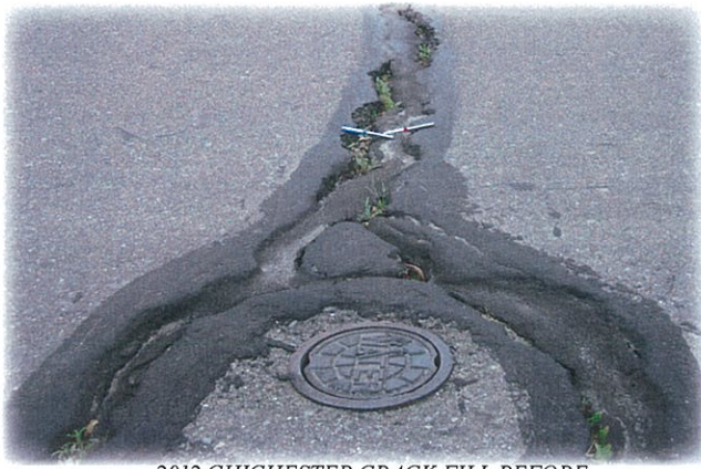
2012 CHICHESTER CRACK FILL BEFORE
