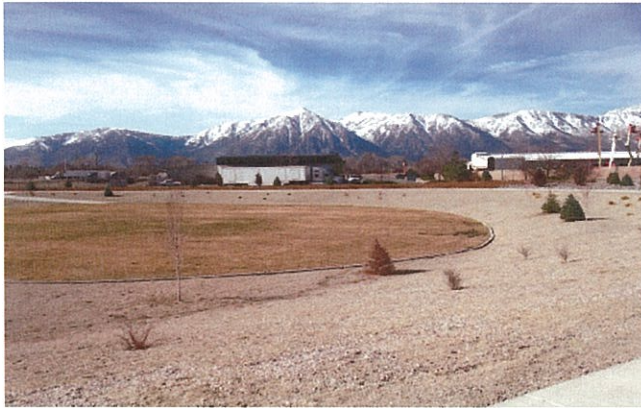
CARRICK/VIRGINIA RANCH DETENTION POND
