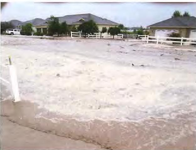
Since the floods of 2014 and 2015, residents have erected property-wide berms to protect their parcels from flooding. These berms have completely altered the natural drainage and were erected without considering the drainage needs of downstream properties. The Johnson Lane ADMP aims to return flows to historic locations and provide regional flood protection.
