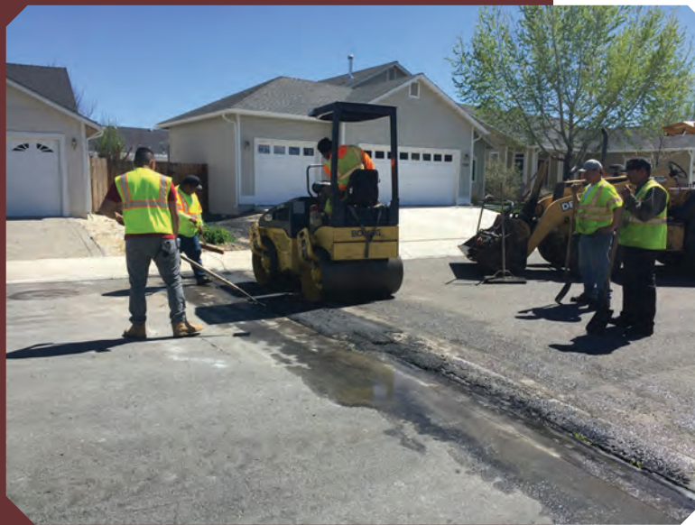
Crack repair
