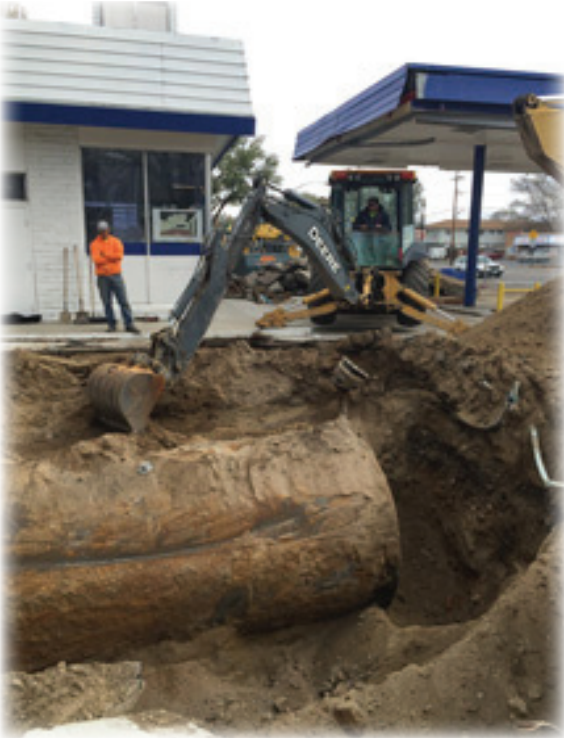
Fuel tank removal
