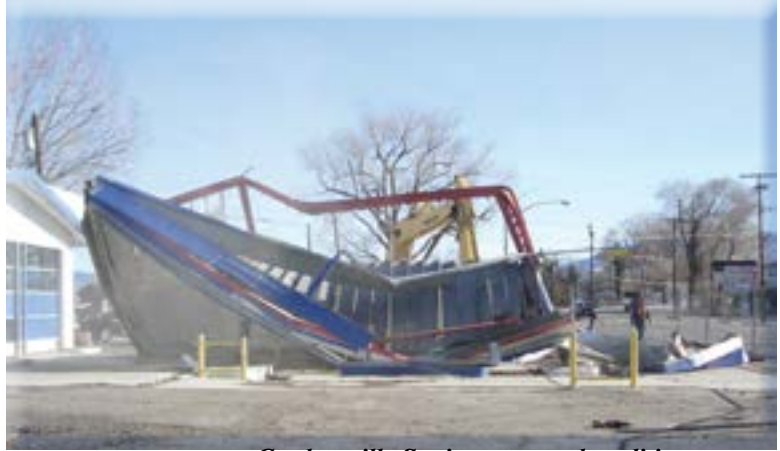
Gardnerville Station canopy demolition
