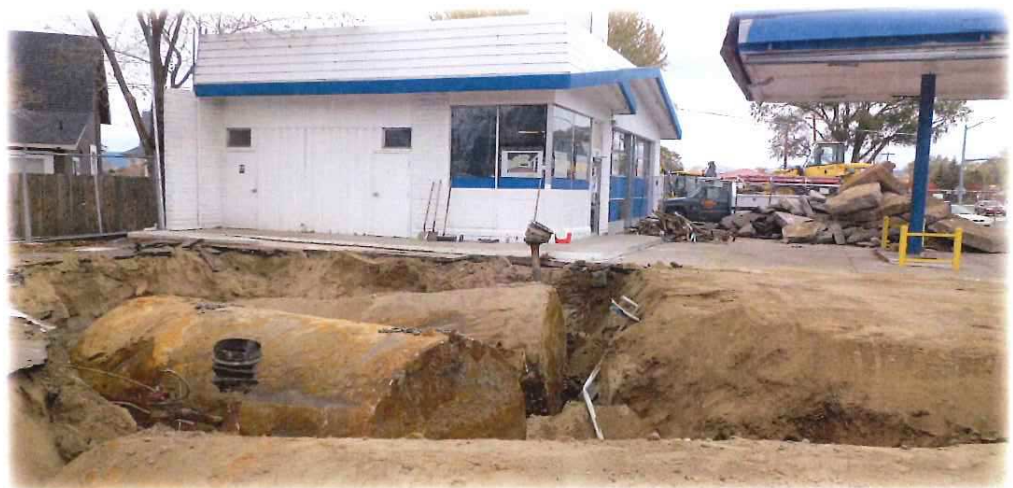
GAS TANKS BEING REMOVED AT GARDNERVILLE STATION
