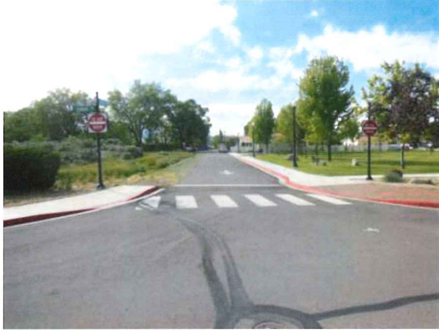
STREET SCENE, LOOKING SOUTHERLY ALONG EZELL STREET, SUBJECT AT LEFT OF PHOTO
