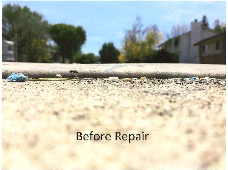
Repair in progress
