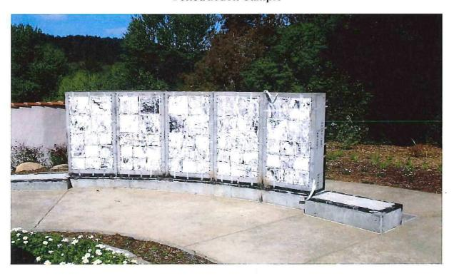
The wall is constructed of concrete and overlaid with granite. Each individual niche has its own Fiberlyte liner and security shutter.
